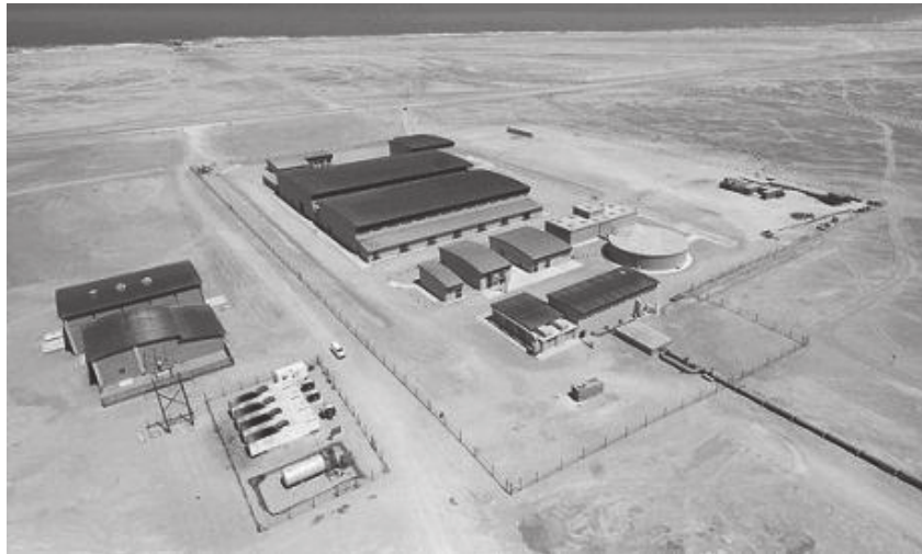
Figure 7: Erongo water desalination plant
